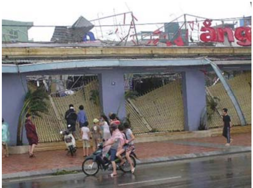
Damage in Da Nang City in Typhoon Xangsane of 2006 (source: Da Nang Center for Flood and Storm Control)
